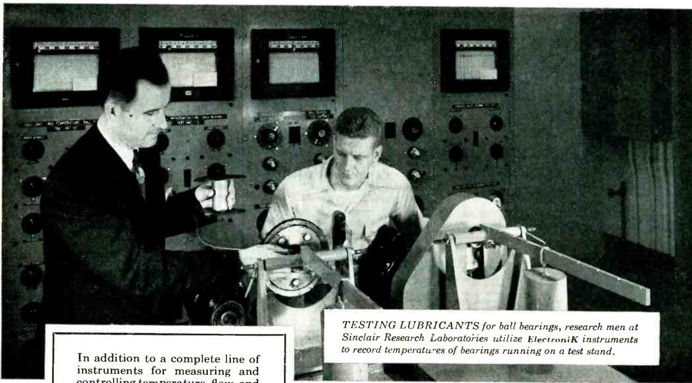
TESTING LUBRICANTS for ball bearings, research men at Sinclair Research Laboratories utilize *ElectroniK* instruments to record temperatures of bearings running on a test stand.
