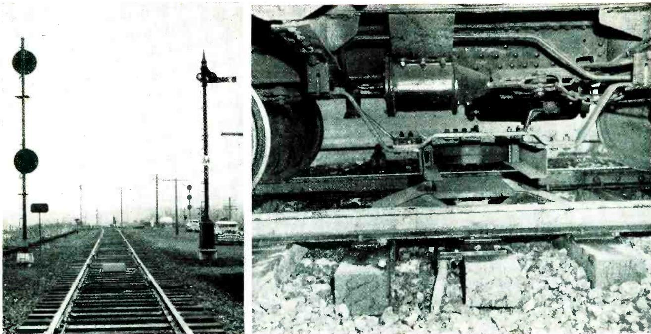
Electronic train identification. Oscillator tank coil in weatherproof housing between tracks couples to tuned circuit in rubber doughnut suspended below caboose, producing change in output
