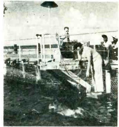
Microphone lowered into tank picks up high frequency sounds emitted by porpoise
