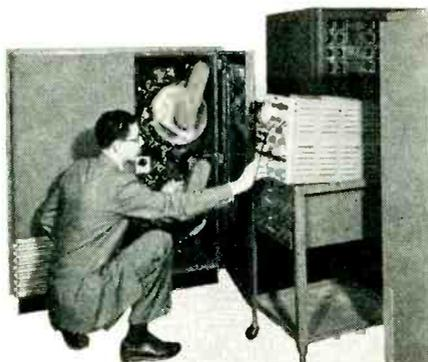
Magnetic Drum Reader and Recorder Unit of the IBM Electronic Data Processing Machines which uses an INDIANA Cunife magnet.
