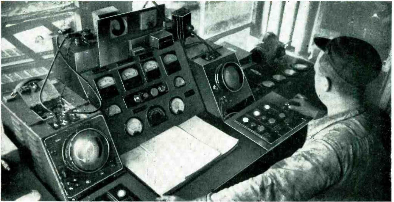
Operator at control station on first floor of mining machine steers cutter along vein by watching pips on two cathode-ray polar-coordinate indicators. Approximately twenty electrical indicating systems, connected to crawler equipment by 57-conductor cable, tell exactly what is going on underground. Operator can steer machine by remote control to mine the desired coal to best advantage, using pips corresponding to bare coal layers and to slate or shale roof and bottom of cut as guides
