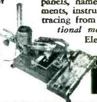
Specify the Green Engraver for precision engraving on metal, plastics, wood, glass, hard rubber etc. . . engraves panels, name plates, scales, dials, molds, lenses, instruments, instruction plates, directional signs . . . by simple tracing from master. Routing, profiling and three dimensional modeling indicate its versatility.
