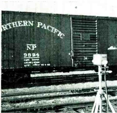
Electronic freight handling. Television camera picks numbers as car enters yard; electronic scales weigh car and record weight
