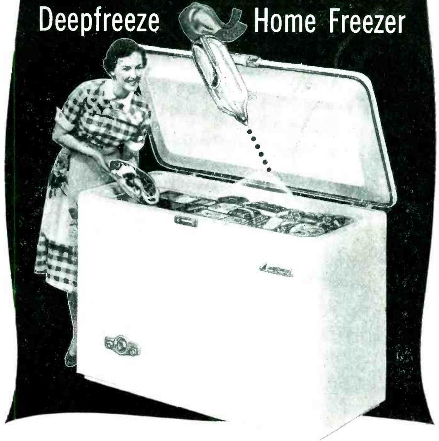
• Hidden in the lid of every Deepfreeze Home Freezer is a Honeywell Mercury Switch. This tiny, glass enclosed unit acts to flash on the lamp which lights up the freezer.
