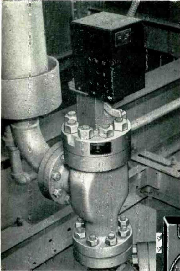
**CONSOLIDATED ELECTROMATIC RELIEF VALVE ACTUATED BY WARD LEONARD RELAYS**, keeps boiler pressures balanced within one percent of a predetermined level. This conserves power, maintains uniform line pressure and decreases maintenance of spring-loaded safety valves.
